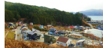
Relocation to upland (Otsuchi Town, Iwate Prefecture)
