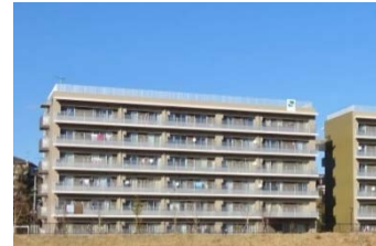
Public housing for disaster-affected people (Ishinomaki City, Miyagi Prefecture)
